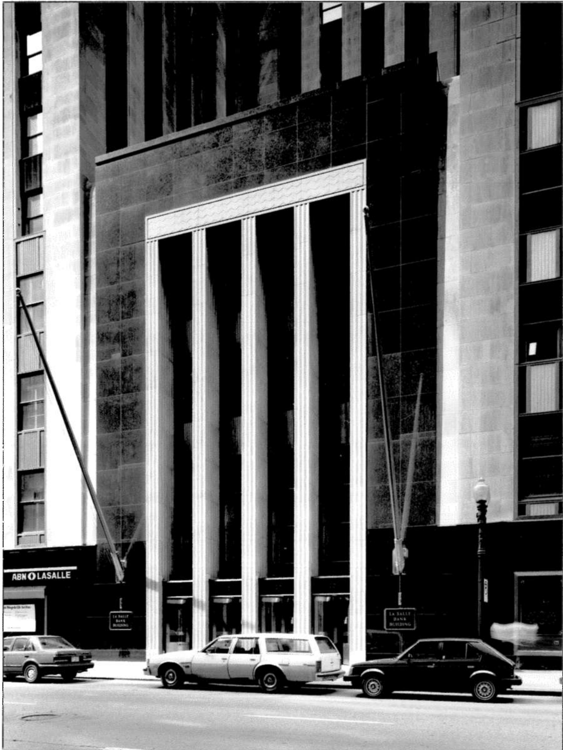
Polished black granite surrounds the dramatically scaled, five-story identical entrances on LaSalle and Clark streets. (Bob Thall, photographer)
